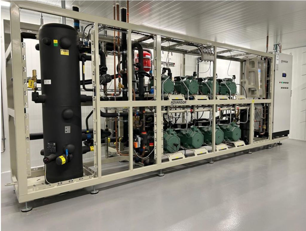
CO2 refrigeration systems provide accurate temperature control
